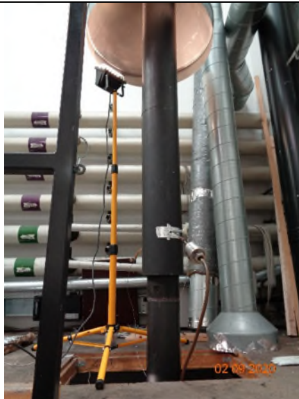
18) Insulated part of the measurement section and the hood. No visible smoke detected.
