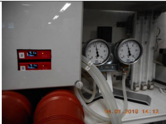
19) Sampling lines flow measurement
